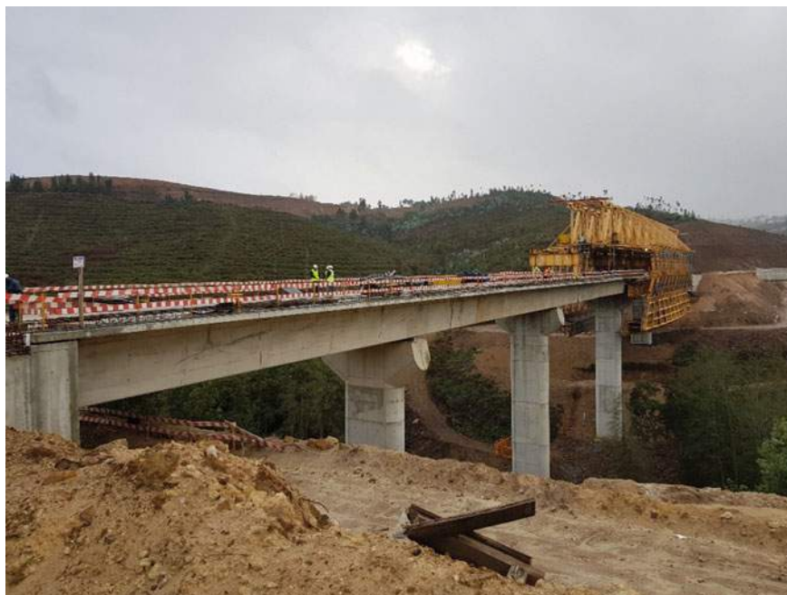
Fig. 1 Bridge over Veade River (personal source, 2020)
